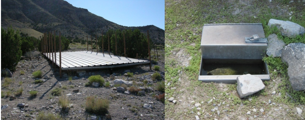
Figure 1. Typical wildlife water development on the Thomas-Dugway Mountains in western Utah, USA, including catchment apron (left) and drinker (right) where we photographed mule deer using water sources, 2007-2011.
